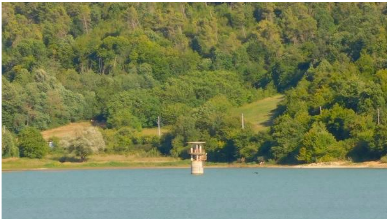
Figure 3: Intake tower; photo by Ermanno De Pisi.
